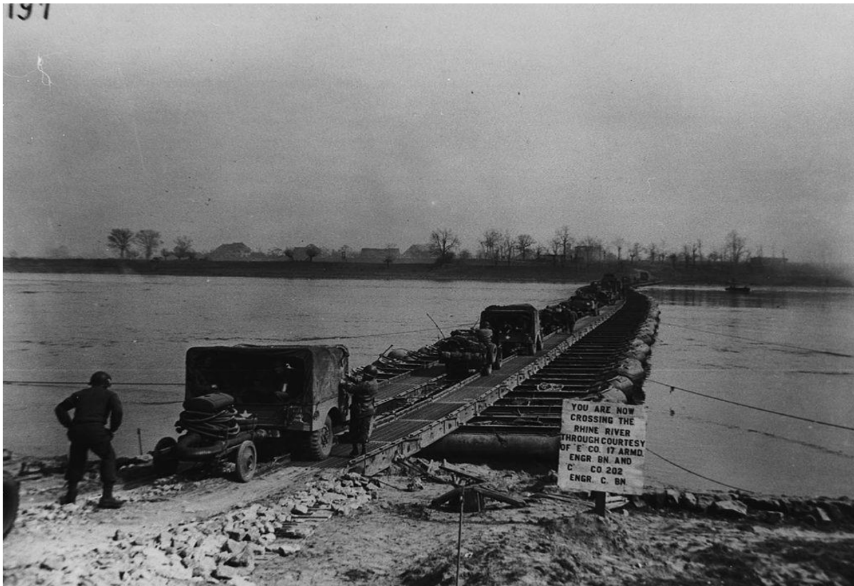
U.S. 9th Army crossing the Rhine River. Wallach. M2, steel treadway, pontoon bridge, late March 1945. Photograph by en.wikipedia.org.
